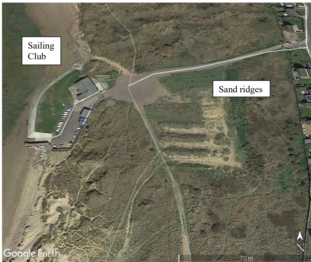
Figure 1a. Aerial photograph of Hightown sand ridges in 2015 (Google Earth).
