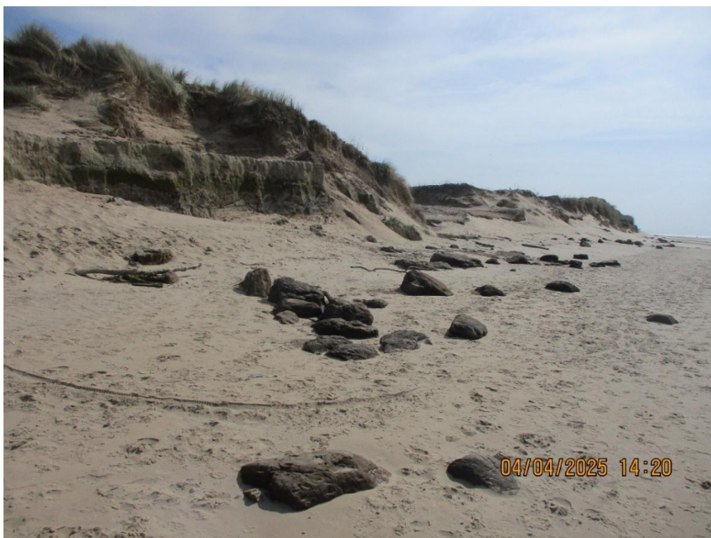
Photograph A3.7 Eroding tobacco waste cliffs near Wick's Lane
