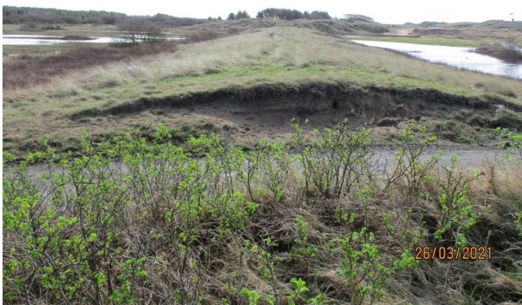
Photograph A3.15 Gap in the bank at cabin Hill
