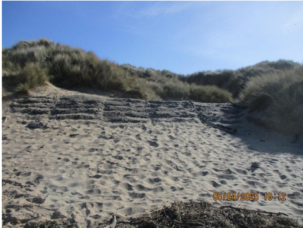
Photograph A4.5 Sloping gabion wall at the northern end of Starr Hills
