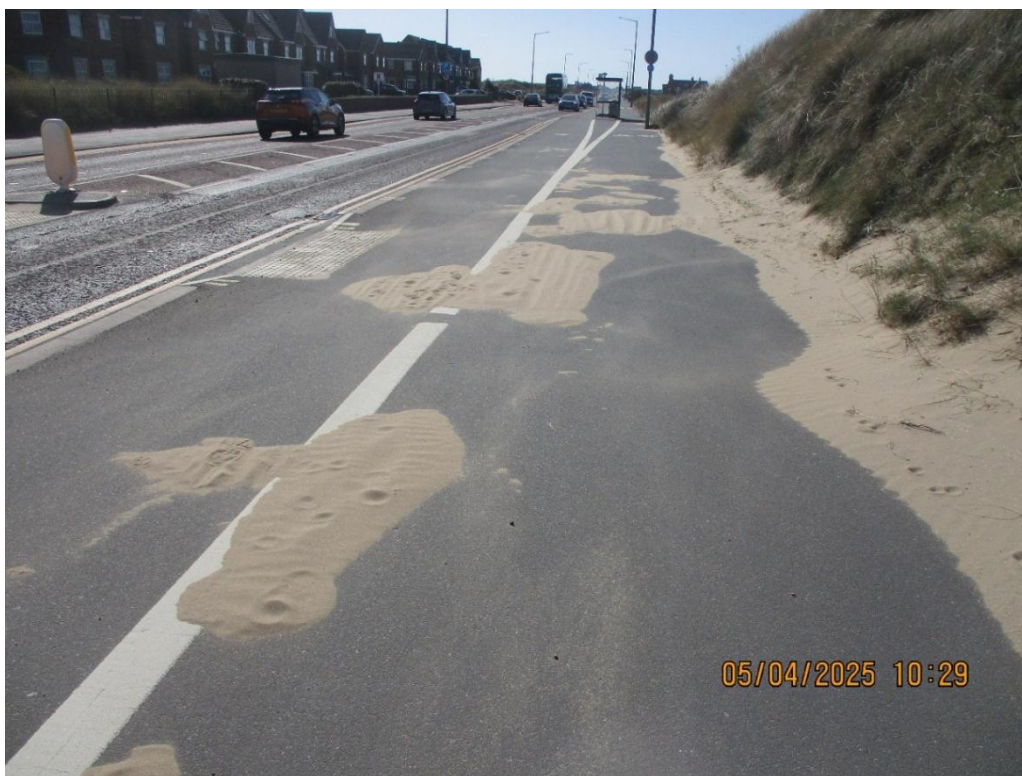
Photograph A4.7 View south along the northern part of Clifton Drive showing mobile sand incursion from degraded dunes to the right
