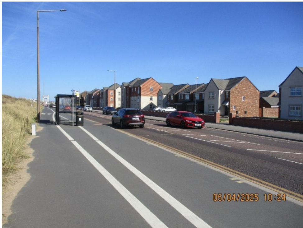
Photograph A4.6 Sand blowing onto the cycleway at the northern end of Cifton Drive; new housing on fomrer Pontins holiday village site to the right
