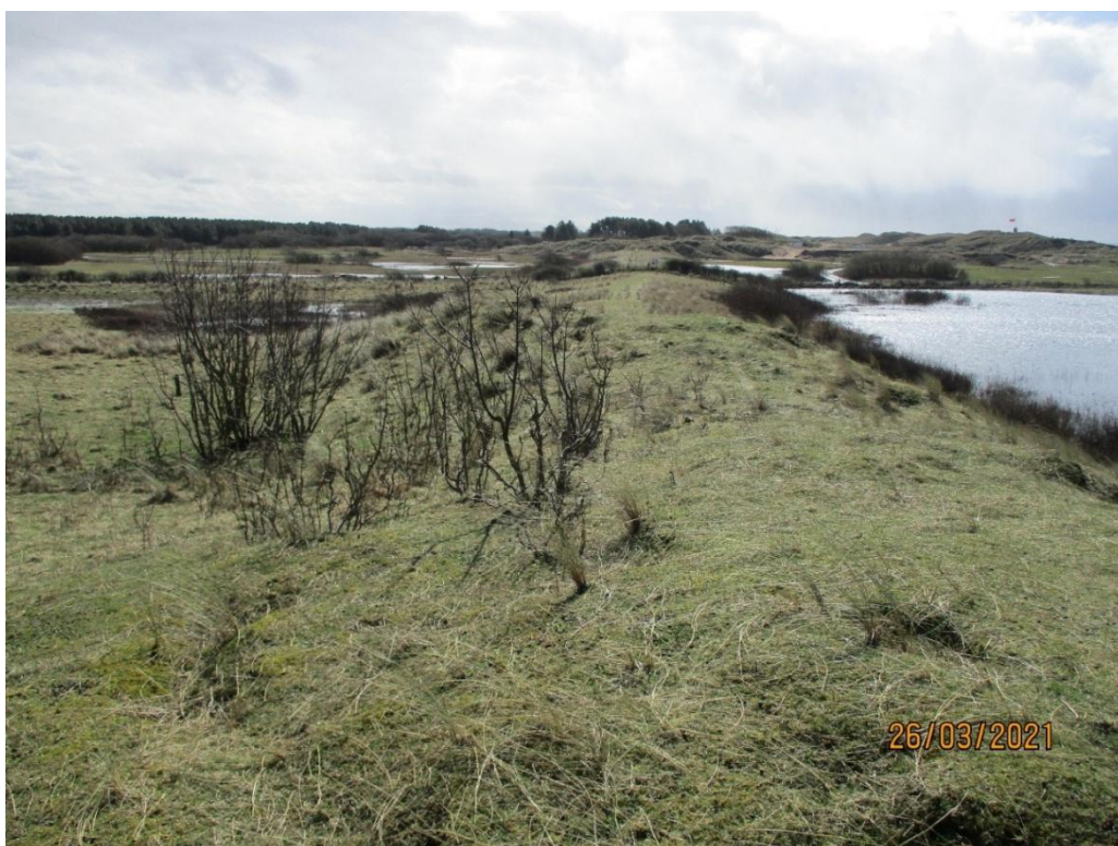
Photograph A3.14 Artificial flood bank at Cabin Hill built in the mid 1970s
