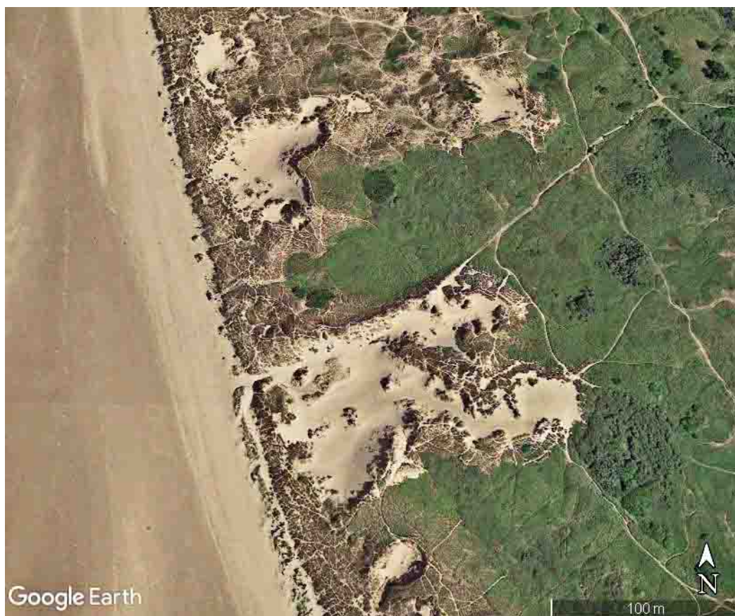
Mobile features at Ravenmeols originating from past sand-winning (Google Earth)
