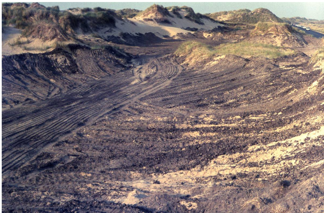
Use of sewage sludge to stabilise sand at Birkdale, 1972
